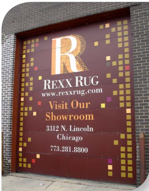
Aluminum panels mounted to garage door
