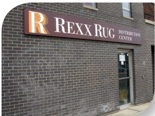
Aluminum panels mounted over entry door
